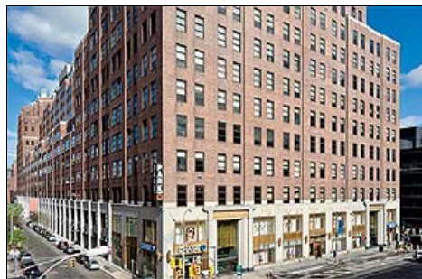
111 Eighth Avenue, which Google purchased for $1.77 billion
